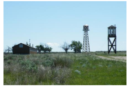
Restored Barracks, Water & Guard Tower
