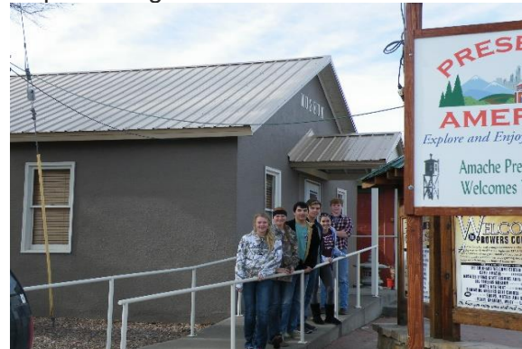
New Roof on the Amache Museum in Granada, CO
