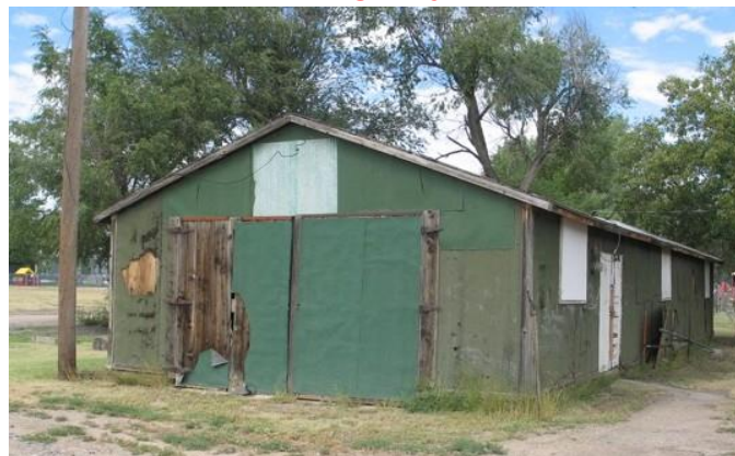
11-F Rec Building in the town of Granada, CO
