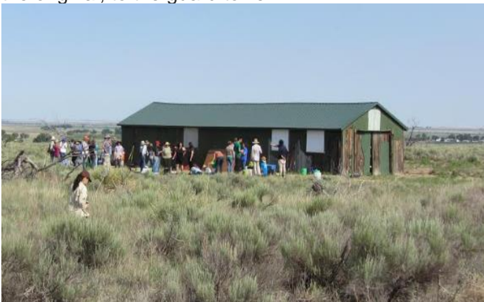
11 F Rec Hall back on its foundation at Amache
